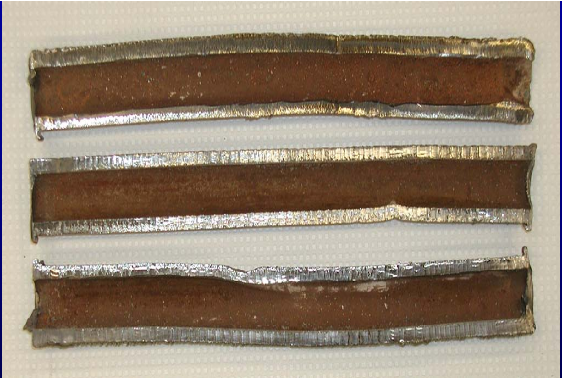
Cut lead service line from D.C. Photo from Mike Schock..
